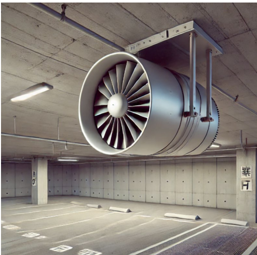
Demonstration of a Jet-Fan
