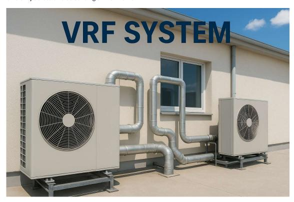
This innovative system architecture features a modular design in which a single outdoor condensing unit, often equipped with advanced inverter-driven compressors, is connected via precisely engineered refrigerant piping to an array of indoor fan coil or ducted units.
