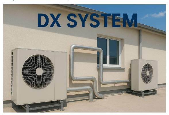
In these systems, a refrigerant evaporator coil is located directly in the air stream that will be supplied to the room; as warm air passes over the cold coil, the refrigerant inside absorbs the heat and expands (changes state from liquid to vapor), thereby cooling the air efficiently. This fundamental process is facilitated by a matched outdoor unit housing a compressor and condenser coil, which rejects the absorbed heat to the outside atmosphere.
