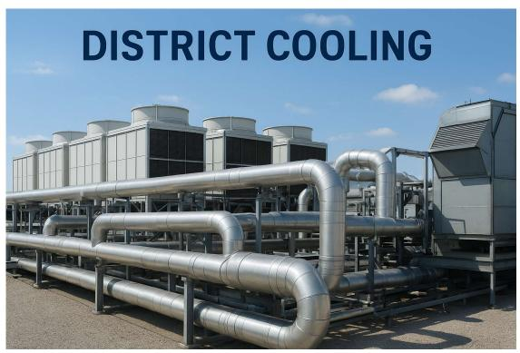
This system utilizes one or more large-scale, water-cooled chillers often equipped with energy-efficient turbocor or magnetic centrifugal compressors and optimized for partial-load performance to generate chilled water at typical temperatures of 4–7°C (39–45°F).
