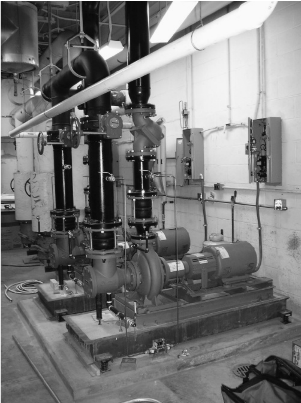
Figure 27.1. PHOTOGRAPH OF FRAME MOUNTED, END SUCTION PUMPS.
