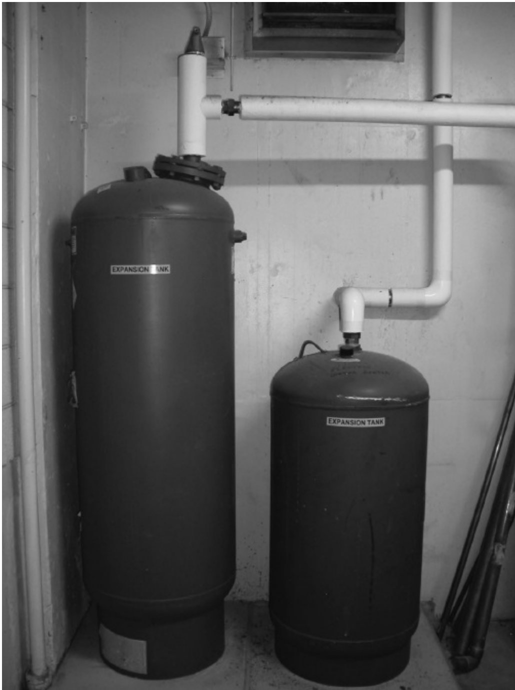
Figure 19.29. PHOTOGRAPH OF AN EXPANSION TANK.
