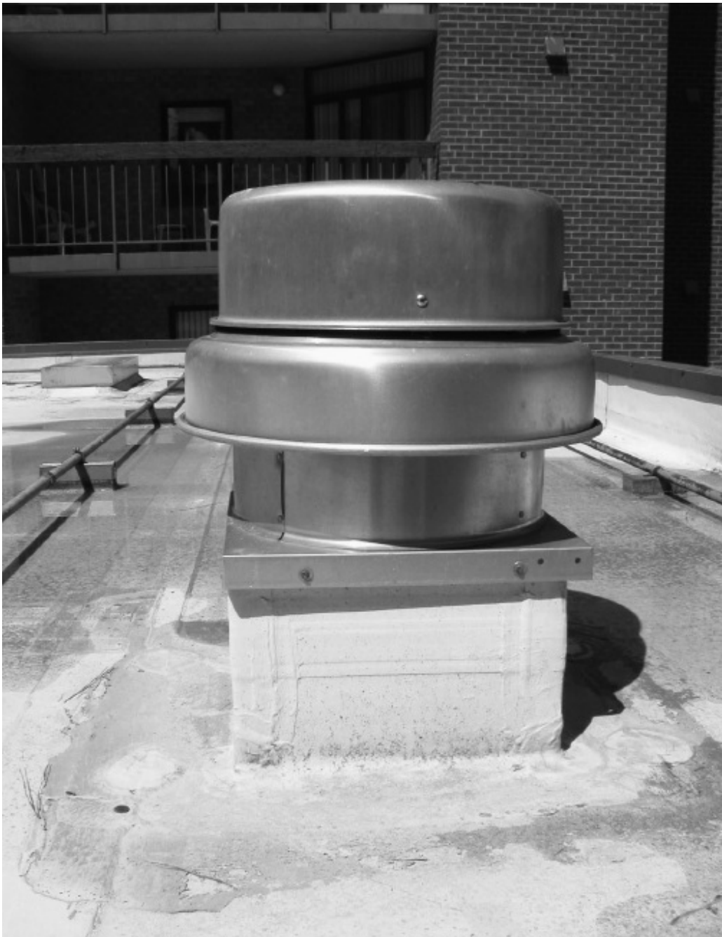
Figure 26.1. PHOTOGRAPH OF A ROOF VENTILATOR.
