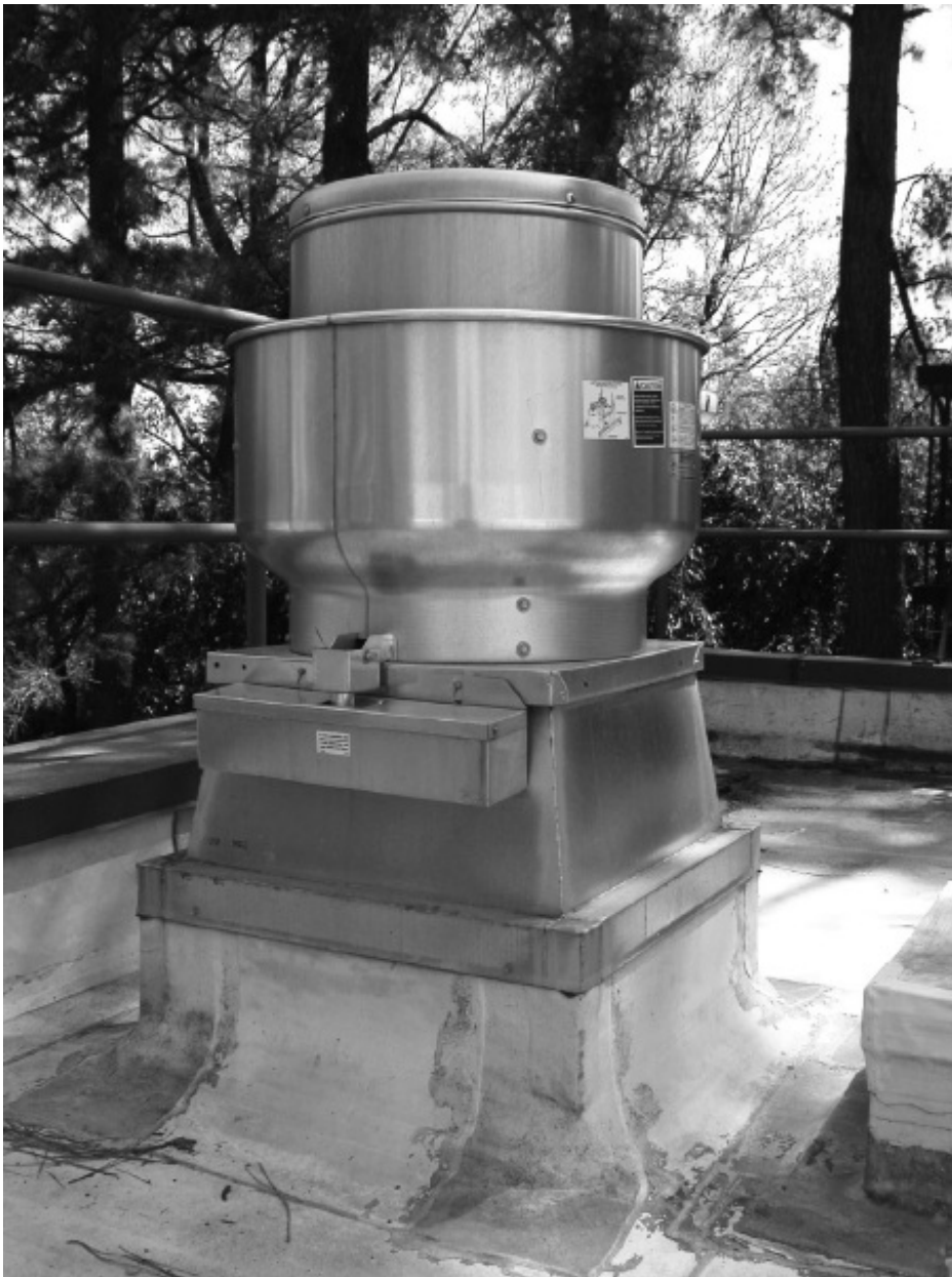
Figure 17.4. PHOTOGRAPH OF AN UPBLAST KITCHEN HOOD EXHAUST FAN.
