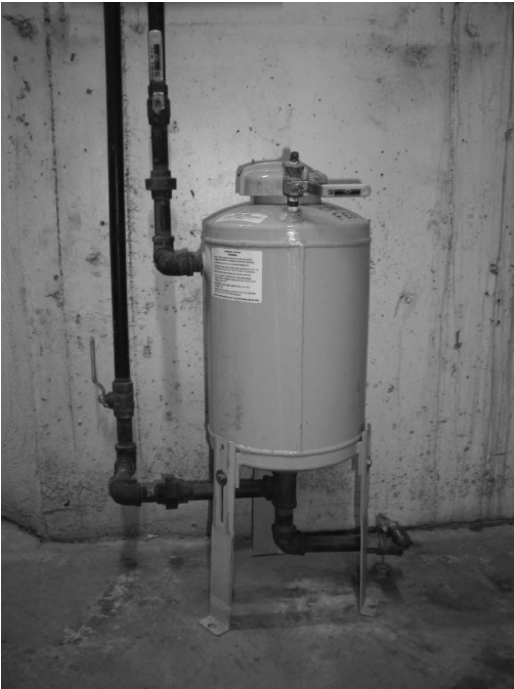
Figure 38.2. PHOTOGRAPH OF A CLOSED SYSTEM CHEMICAL SHOT FEEDER.
