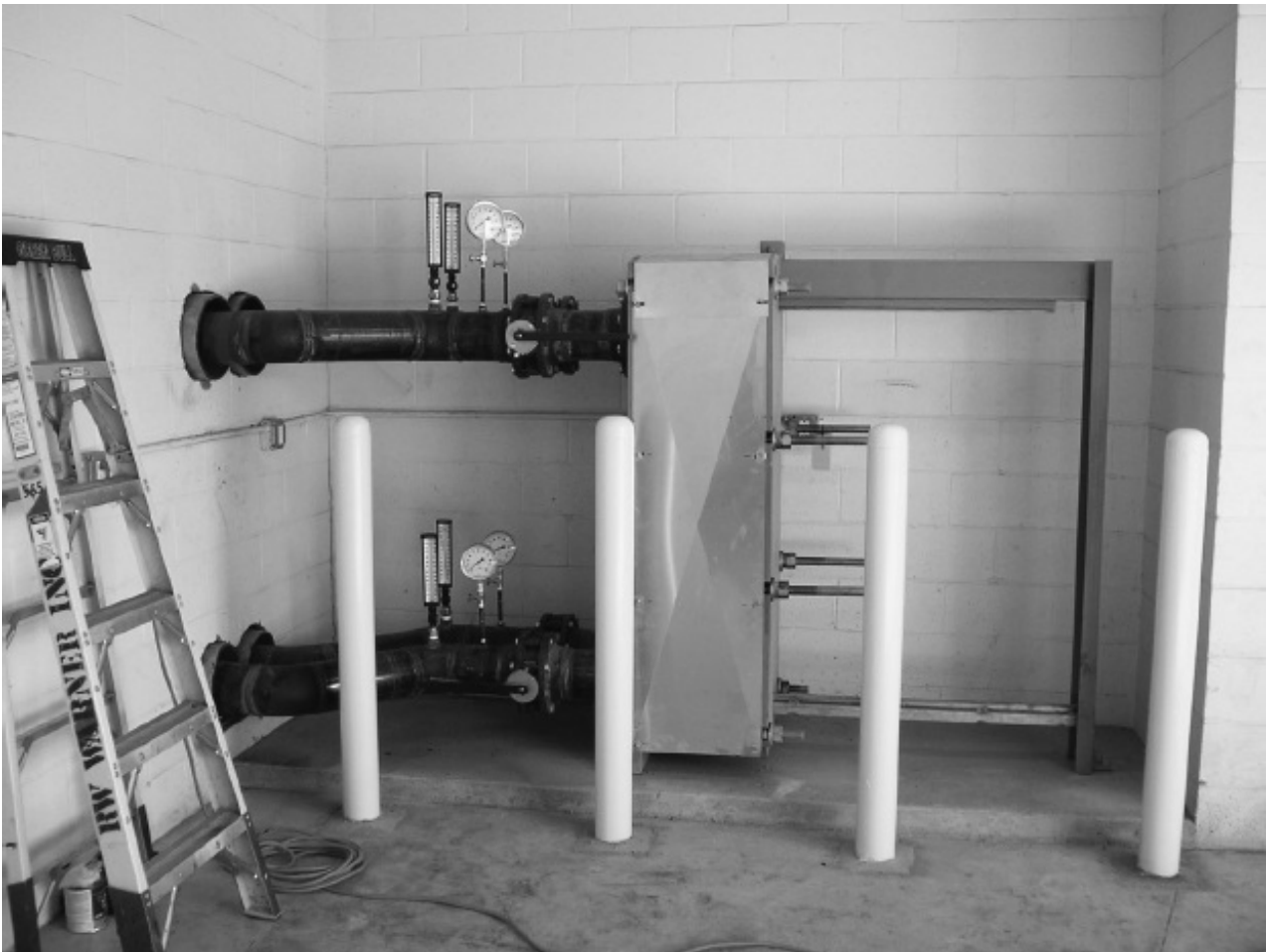
Figure 30.1. PHOTOGRAPH OF A PLATE AND FRAME HEAT EXCHANGER.
