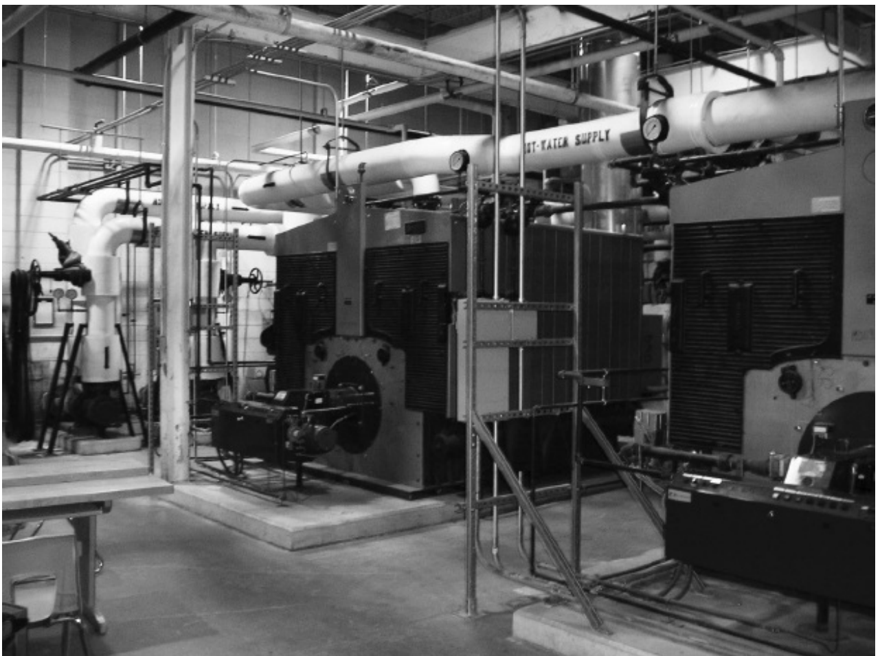
Figure 31.4. PHOTOGRAPH OF WET BASE CAST IRON BOILER.
