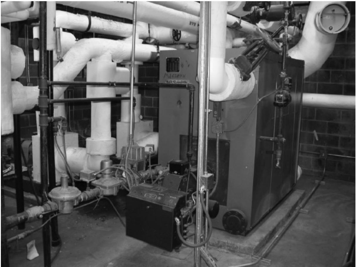
Figure 31.4. PHOTOGRAPH OF WET BASE CAST IRON BOILER.
