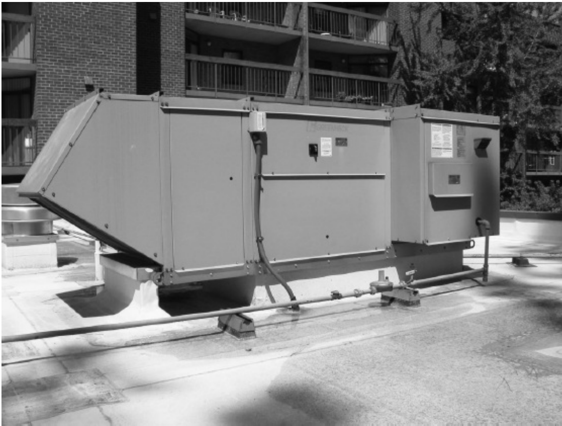
Figure 17.5. PHOTOGRAPH OF A KITCHEN HOOD MAKEUP AIR UNIT.
