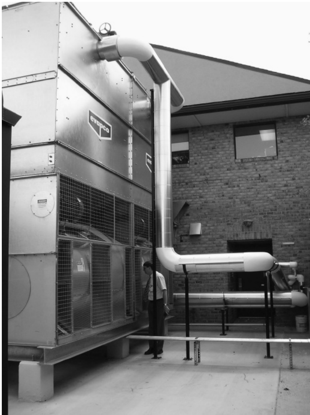
Figure 29.1. PHOTOGRAPH OF A FORCED DRAFT, COUNTER FLOW COOLING TOWER.
