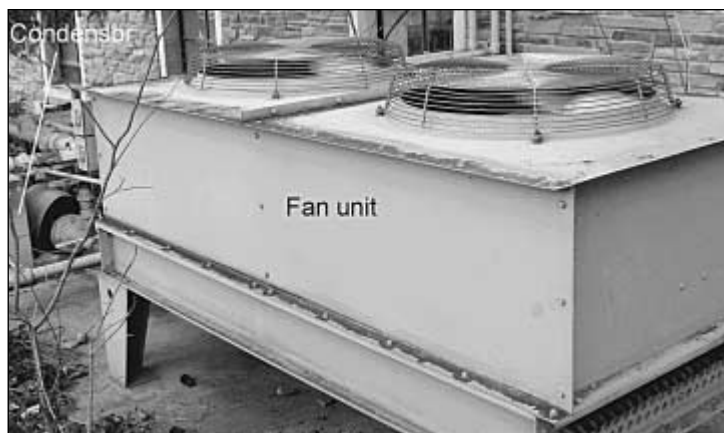
FIGURE 9.4 Dry cooler.
