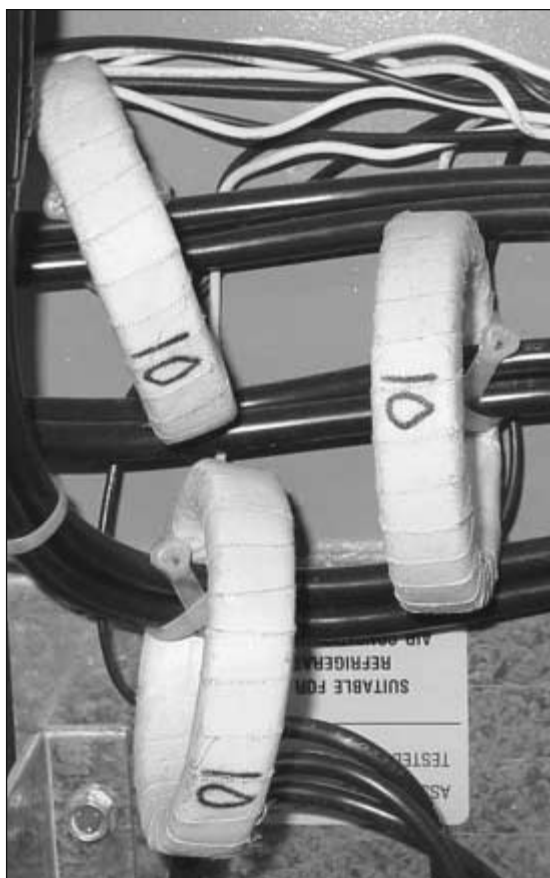
FIGURE 5.28 Solid-core current transducers.
