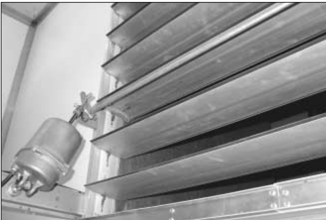
FIGURE 13.5 Pneumatic actuator on tight-seal outdoor air dampers.
