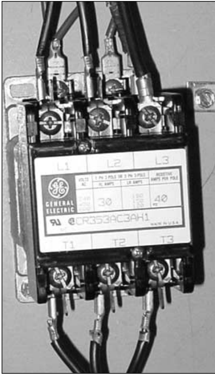
FIGURE 4.21 Three-phase contactor.
