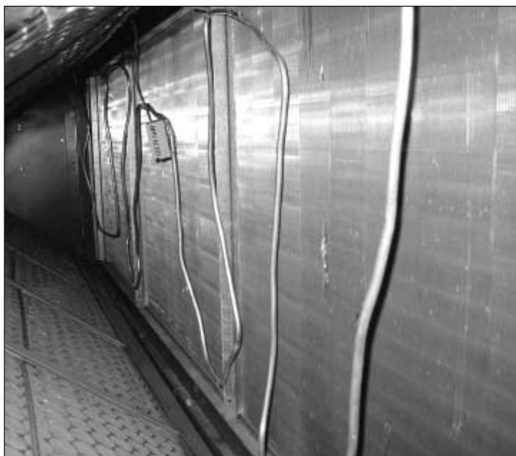
FIGURE 5.10 Duct averaging RTD sensor.
