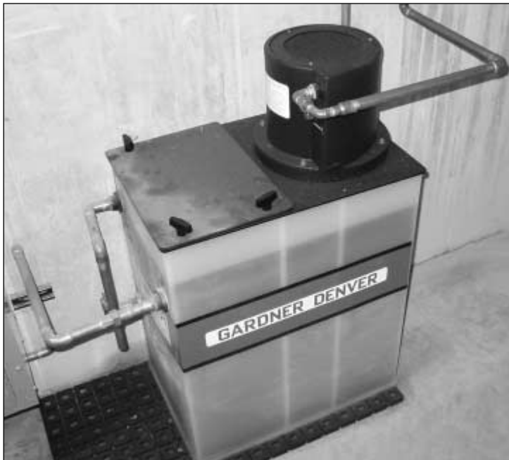
FIGURE 2.16 Water/oil separator.
