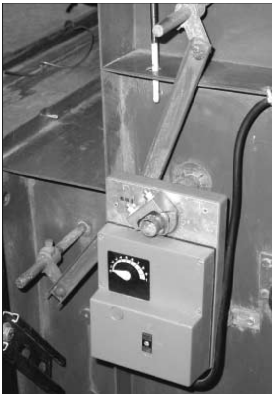
FIGURE 5.41 Electronic damper actuator and linkage.
