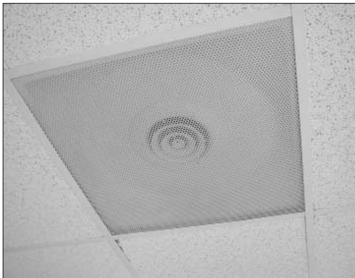
FIGURE 16.9 Zone air diffuser.
