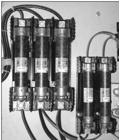
FIGURE 4.18 Fuse bank.
