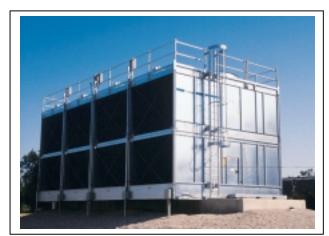
Forced draft towers have fans on the air inlet to push air either counterflow or crossflow to the movement of the water. Forward curved fans are often employed. They use more fan power than induced draft but can provide external static pressure when required. This can be important if the cooling tower requires ducting, discharge cap or other device that creates a pressure drop.
